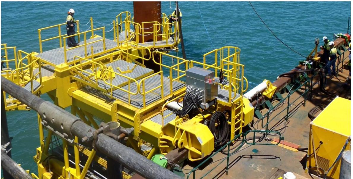
*Piling template at Hay Point during pile driving*
