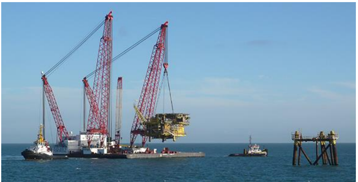
Decommissioning of topside and jacket of Camelot platform
